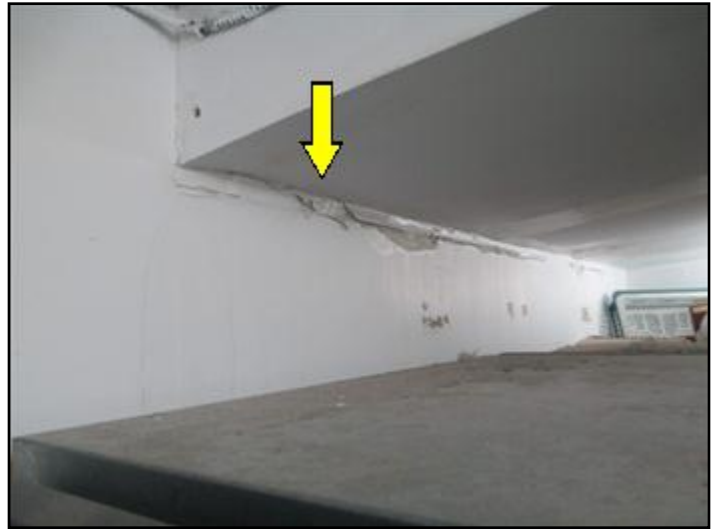
Water damage at rear junction storage room
