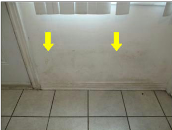
Problems visible with rear wall # 3
