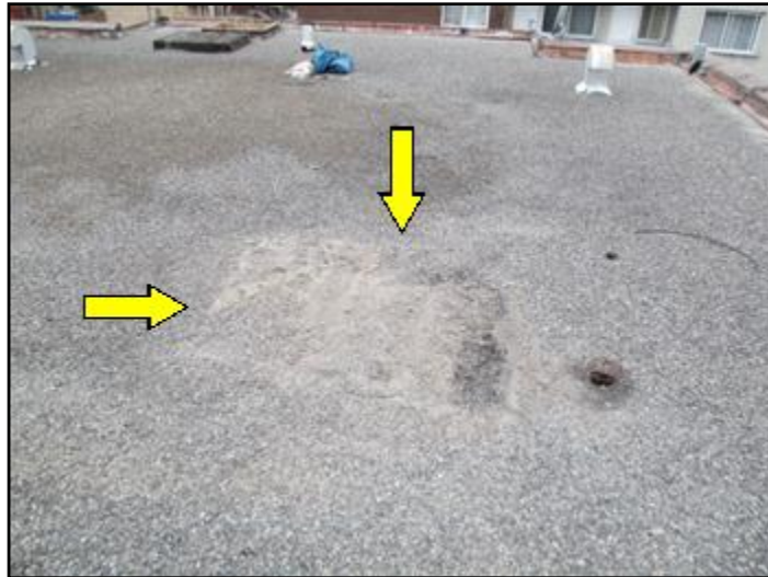
Roof patch visible near drain
