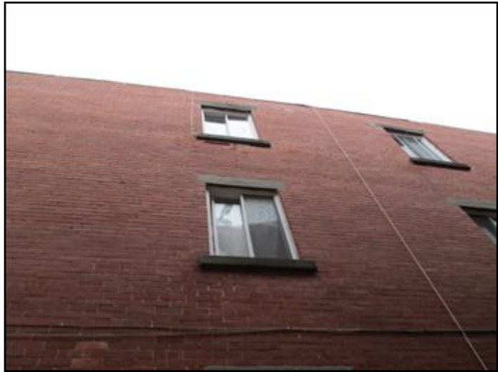
Bowing and waves of third floor masonry
