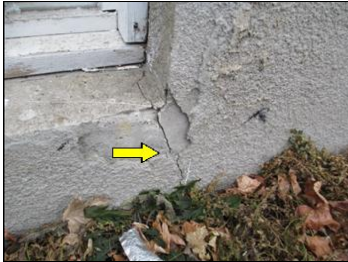
Foundation crack in left wall
