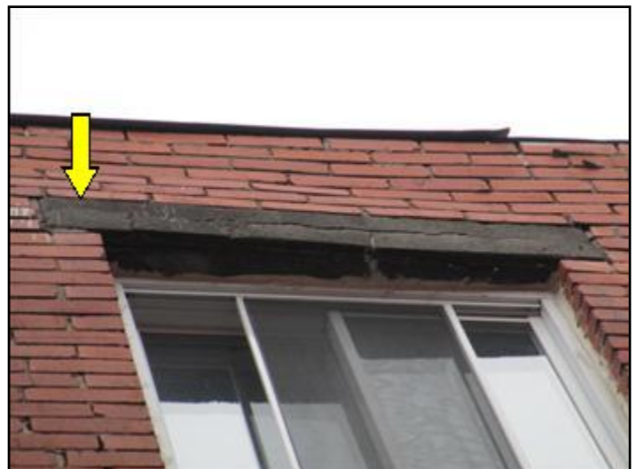
The lintel is pulling away from the building
