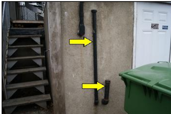
Oil fill pipes on left exterior wall at rear
