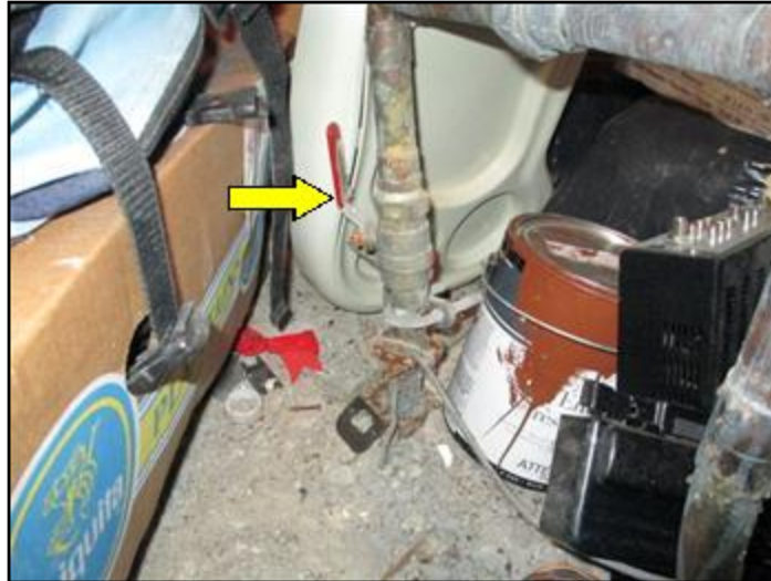
Water main for building under front entrance
