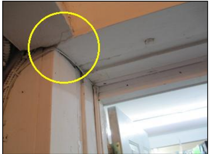
Water stains at rear junction storage room
