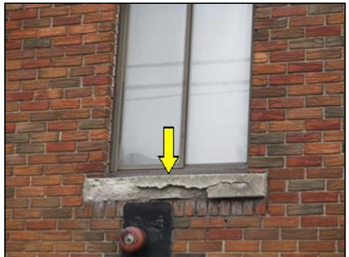
Deteriorated window sill left wall
