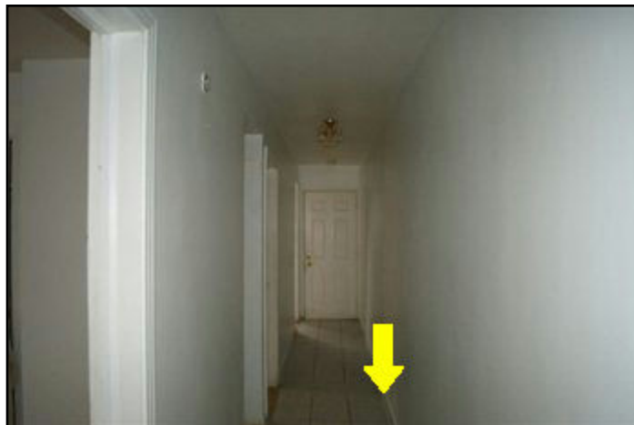
Floor sloped towards center wall in apt 7
