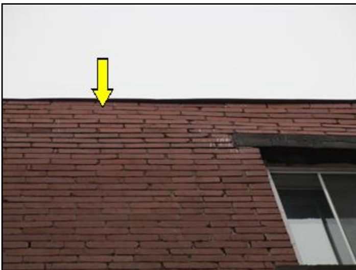
A bulge has appeared in top section of wall
