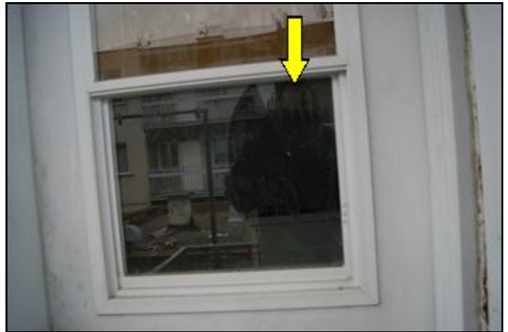
Broken glass pane at rear
