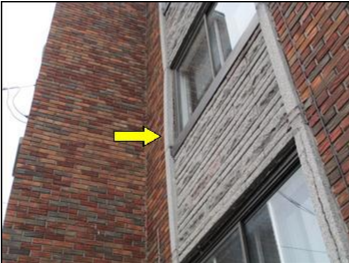
Pre-cast masonry pulling away
