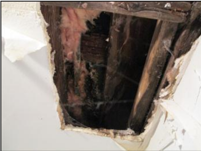
Roof support weakened by prior water infiltra
