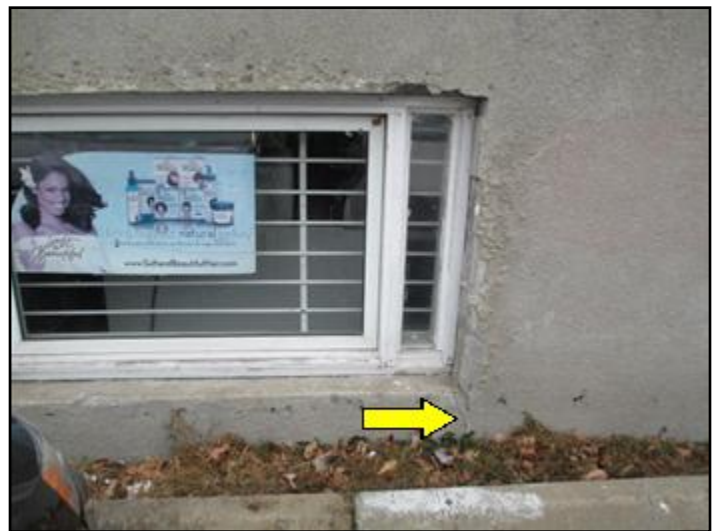
Foundation crack in left wall
