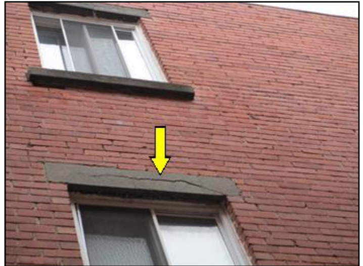
Cracked window lintel right wall
