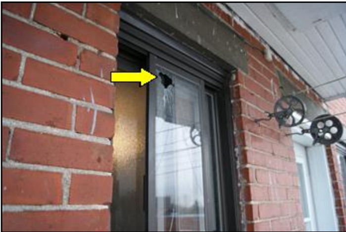
Broken glass pane at rear
