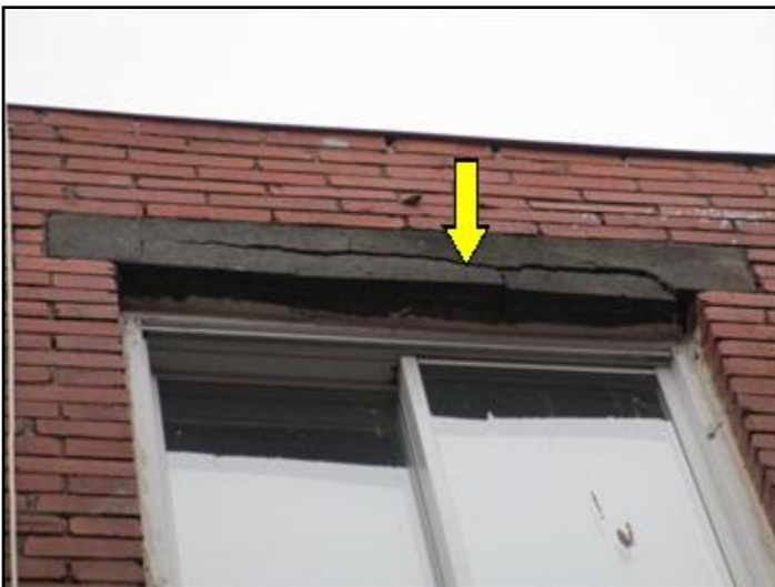
Cracked window lintel right wall
