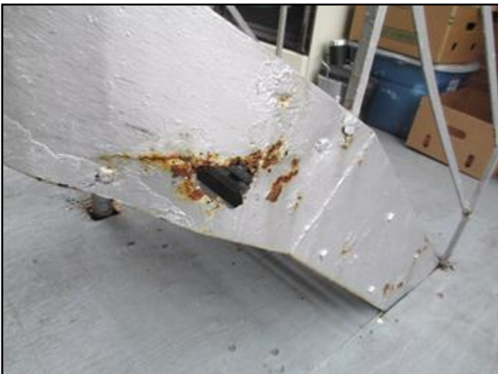
Rear fire escape stairs are severely corroded
