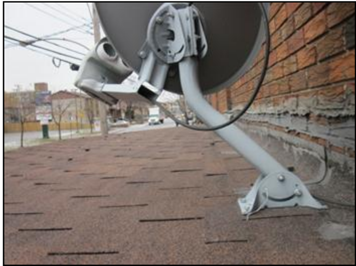
Shingles installed on low slope roof
