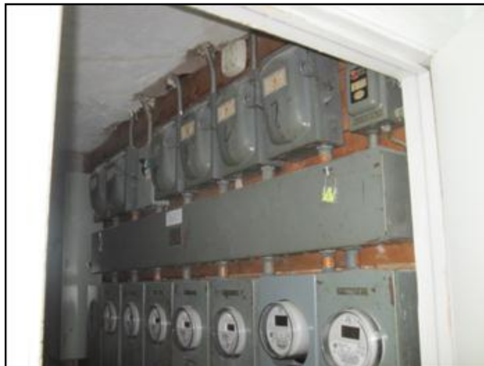
Main electrical room at top of third floor
