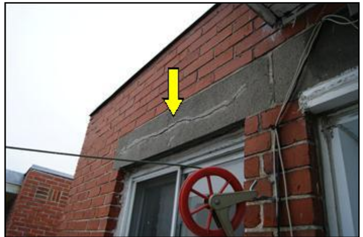
Cracked window lintel rear wall
