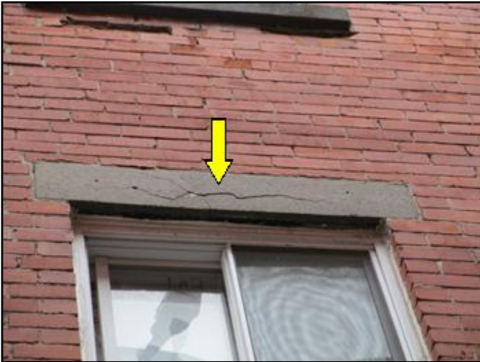
Cracked window lintel right wall
