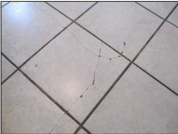
Cracked ceramic tiles in apt 5
