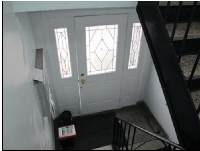
Missing heater in front staircase
