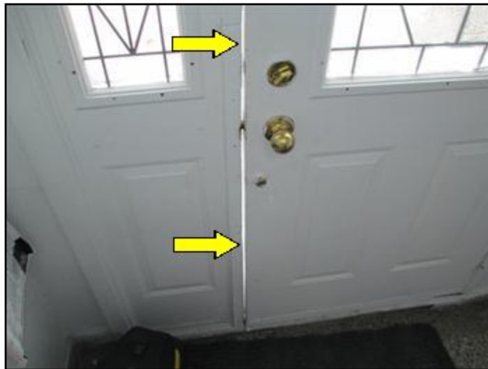
Significant air leakage around front door
