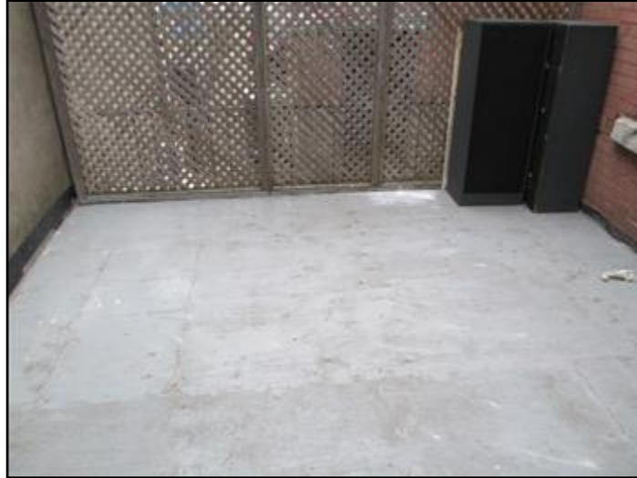
Secondary roof at rear covered by wood deck
