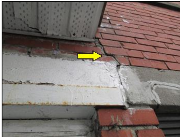
Crack in rear masonry wall
