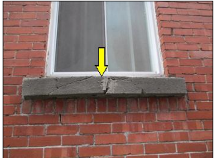
Deteriorated window sill right wall
