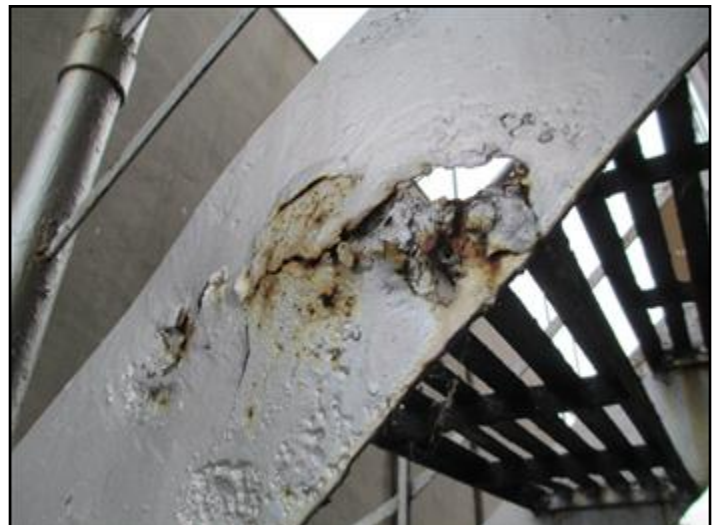
Rear fire escape stairs are severely corroded
