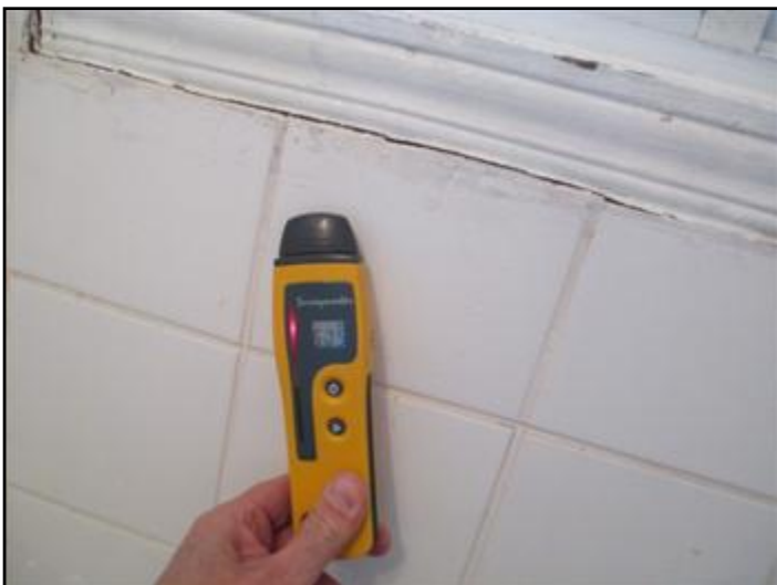
High moisture level detected in apt #6
