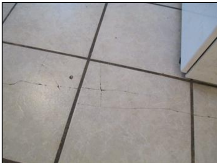
Cracked ceramic tiles in apt 5
