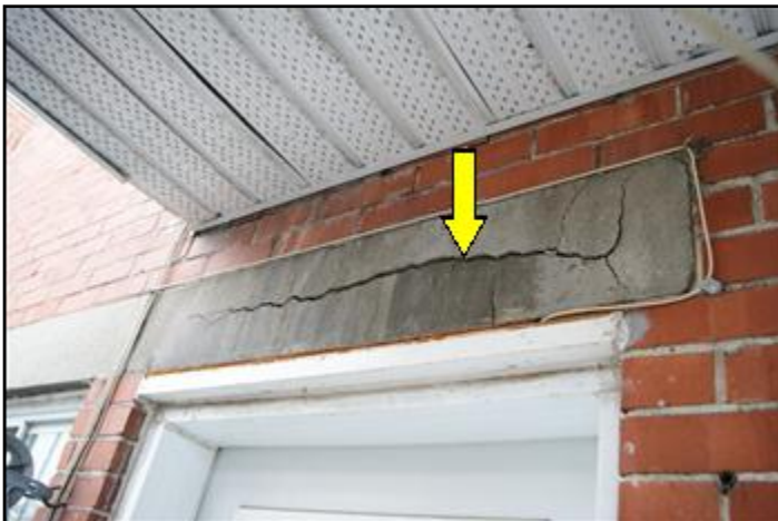
Cracked window lintel rear wall
