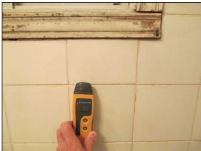
High moisture level detected in apt #4
