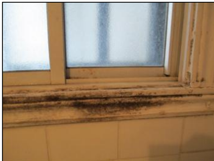
Appearance of mold in bathroom of apt 2
