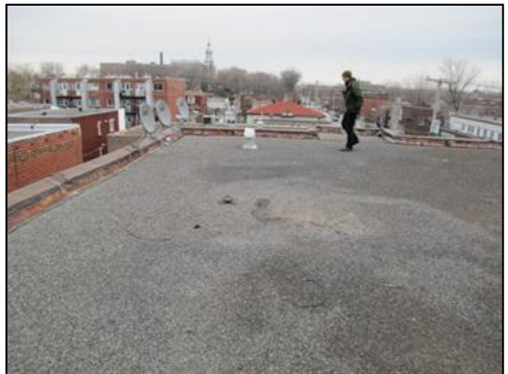
Partial view of roof towards the front
