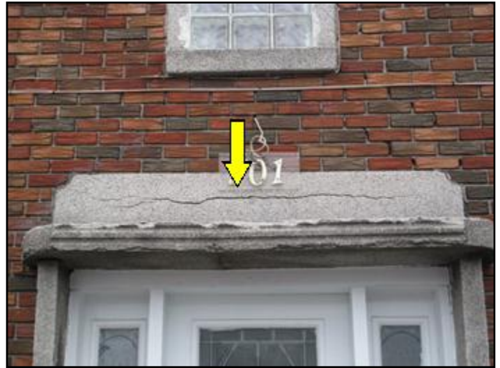
Pre-cast masonry cracked
