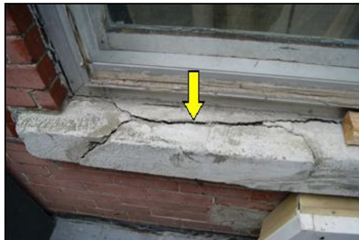
Cracked window sill rear wall
