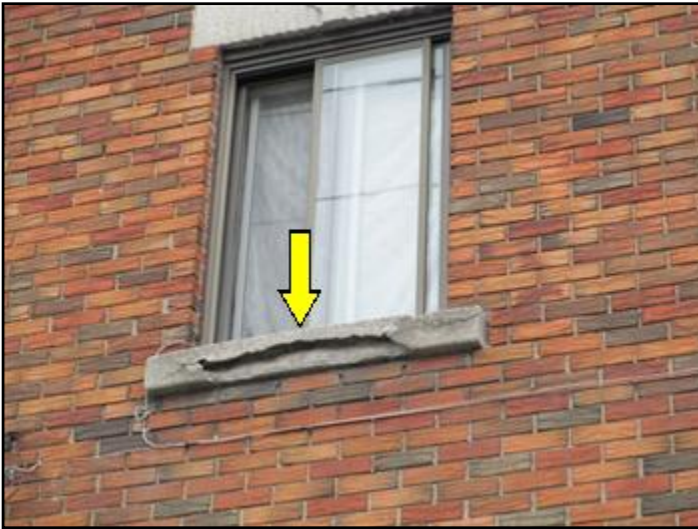
Deteriorated window sill left wall
