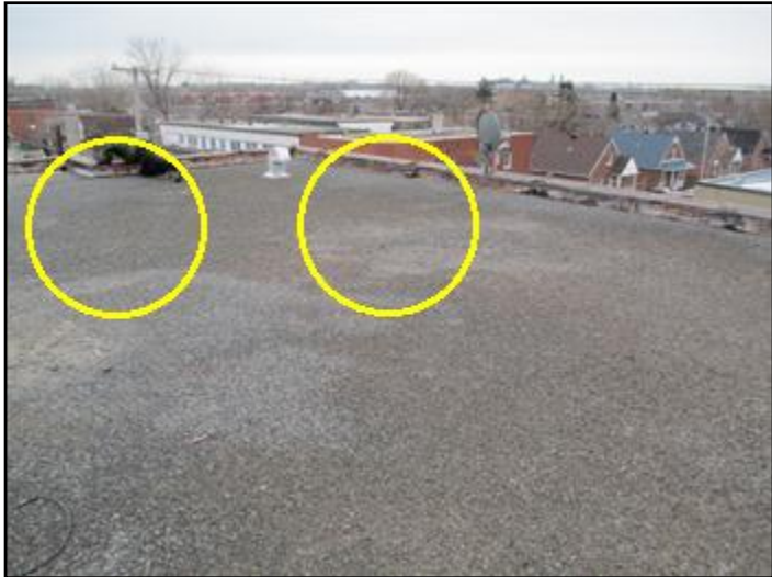
Symptoms of water ponding visible
