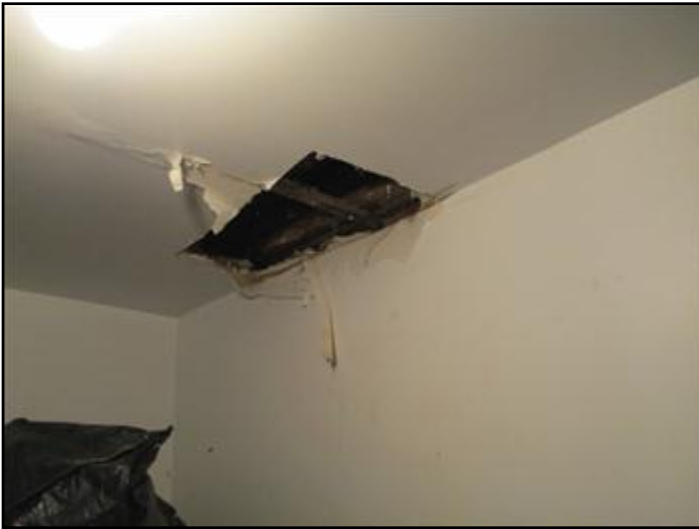
Water infiltration in right rear storage
