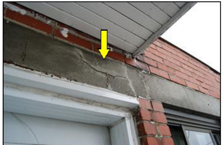
Cracked window lintel rear wall
