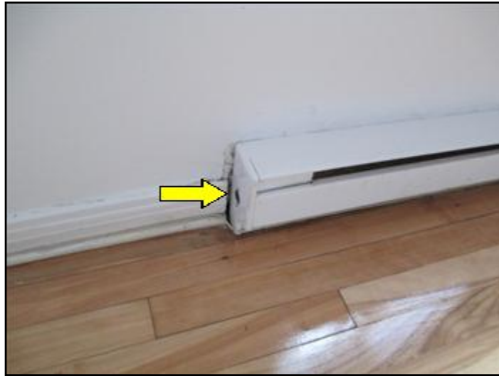
Control knob missing in bedroom of apt 7
