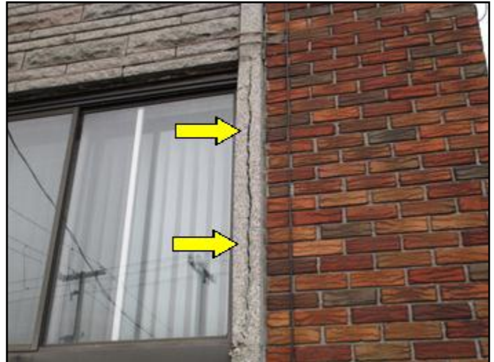
Pre-cast masonry cracked
