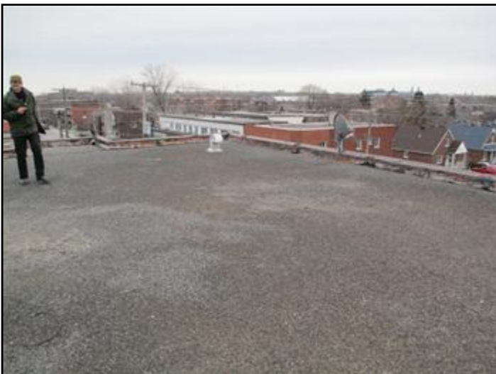
Partial view of roof towards the front
