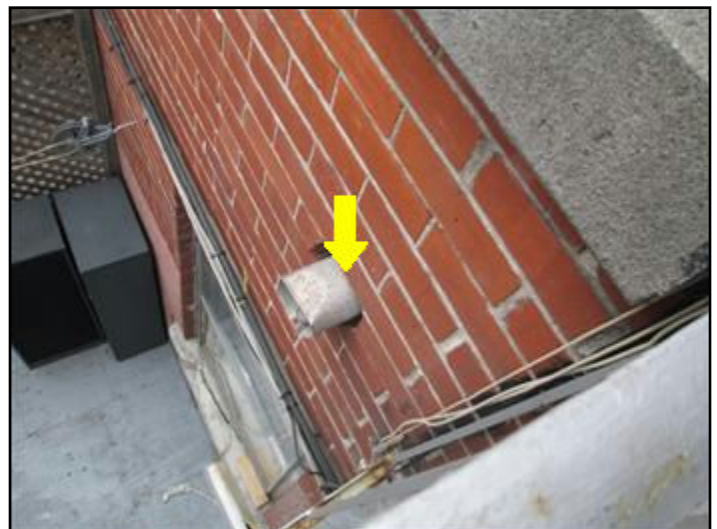
Weather hood missing or loose
