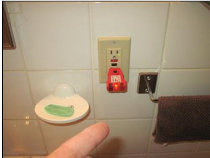
Bathroom outlets not grounded
