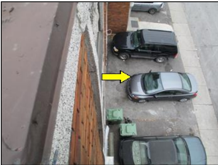
Pre-cast masonry pulling away
