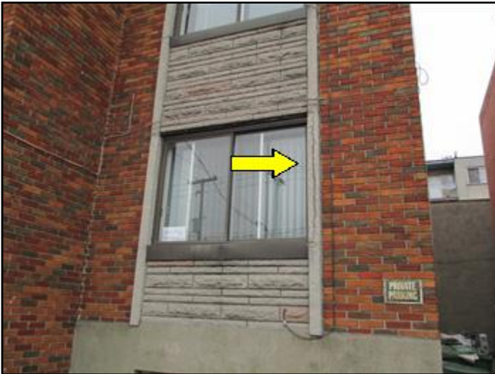
Pre-cast masonry cracked
