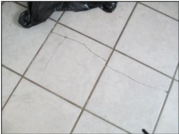
Cracked ceramic tiles in apt 4
