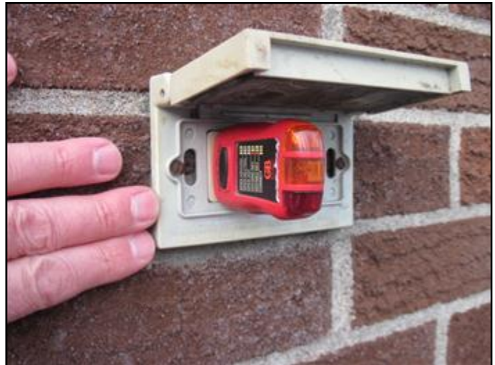
Open neutral condition detected
