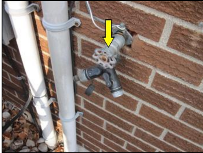
Backflow missing on hose bibb
