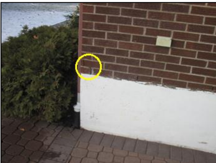
Crack in left brick wall rear corner
