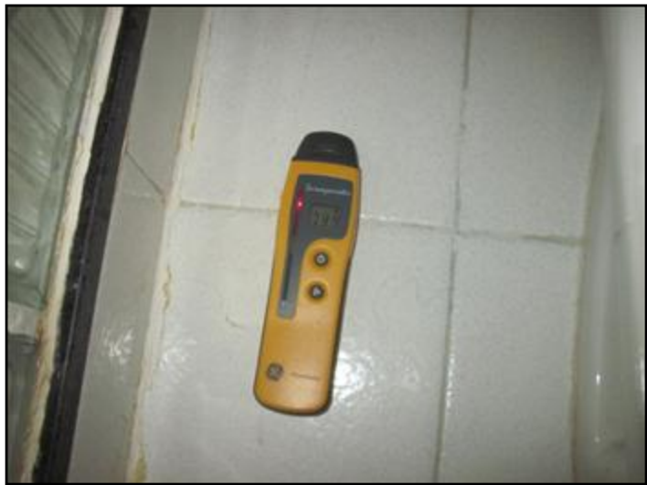
High moisture level detected under ceramic
