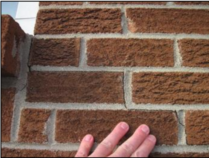
Crack in left brick wall middle section
