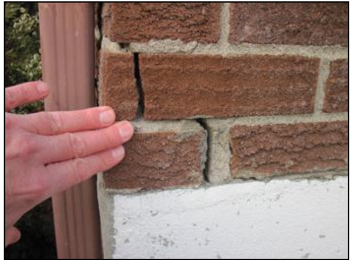
Crack in left brick wall rear corner
