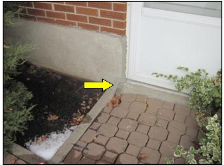
Crack in rear garage wall
