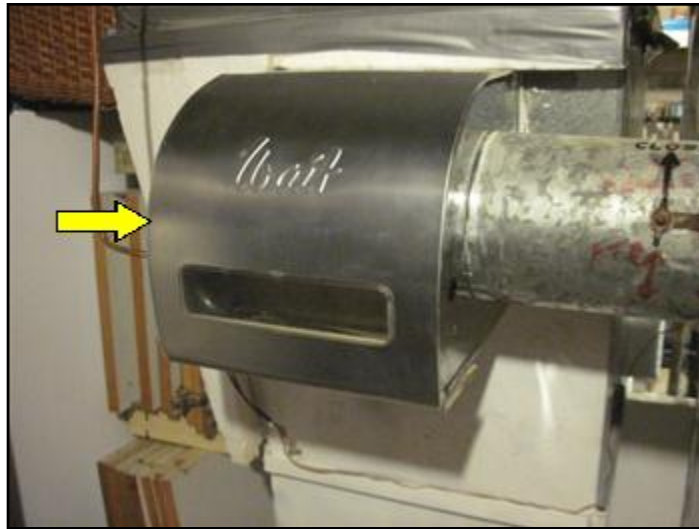
Clean drum humidified regularly
