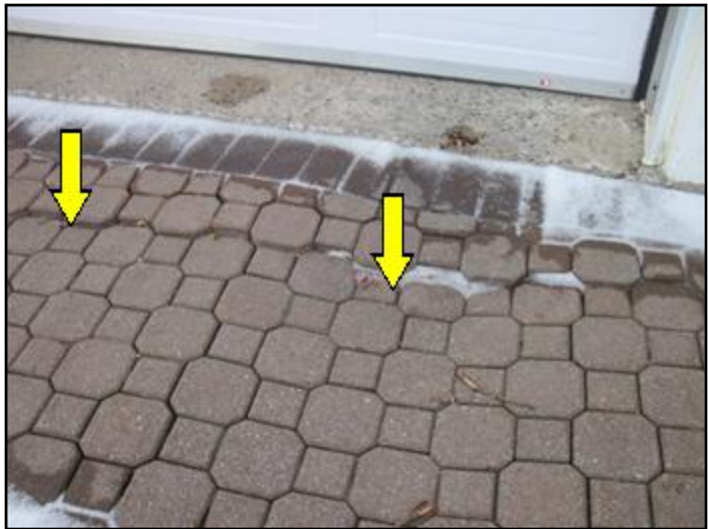
Excessive settlement in driveway
