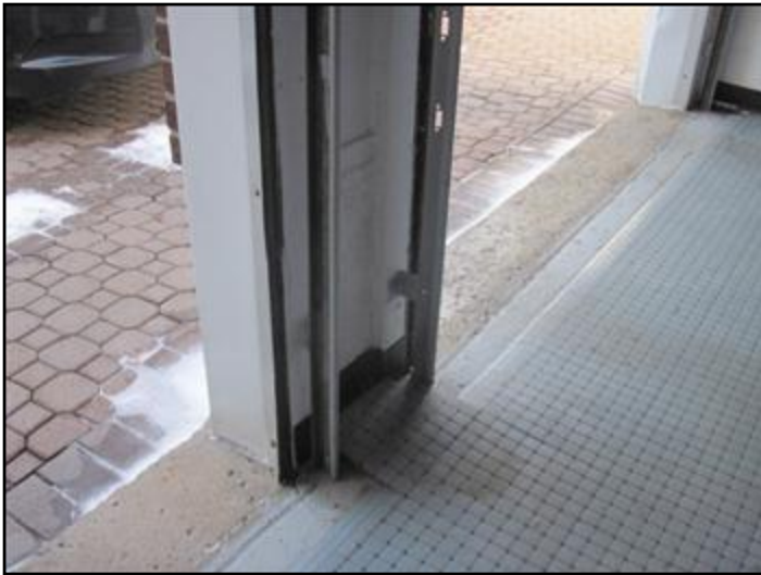
Infrared sensors missing on GDO's
