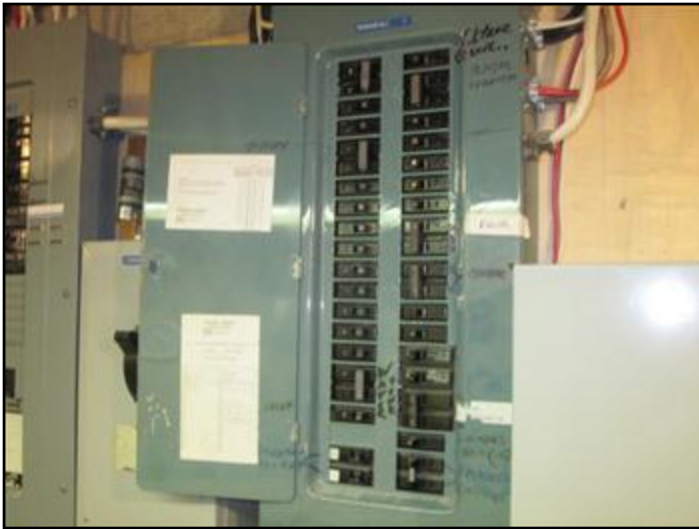
Crouse Hinds Breaker Panel
