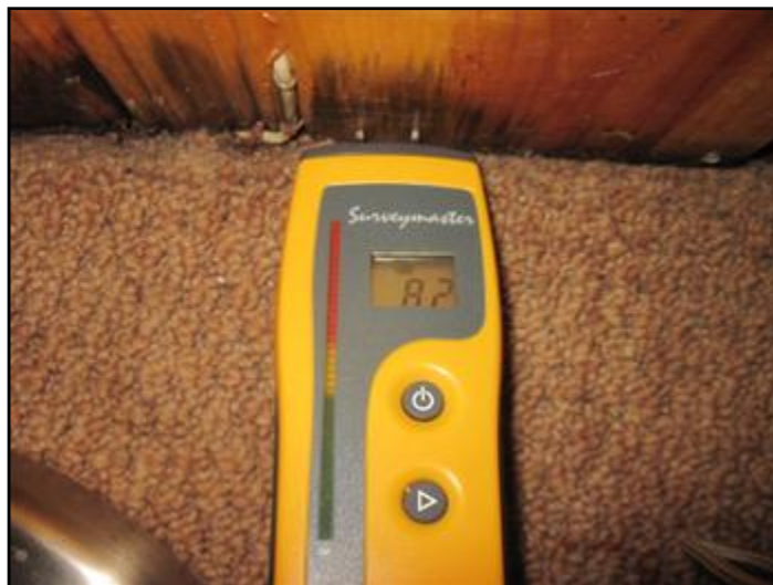
Testing for moisture in basement
