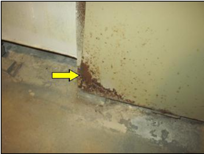
Rust exterior furnace cabinet
