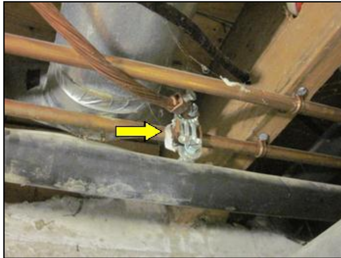
Inappropriate ground connection
