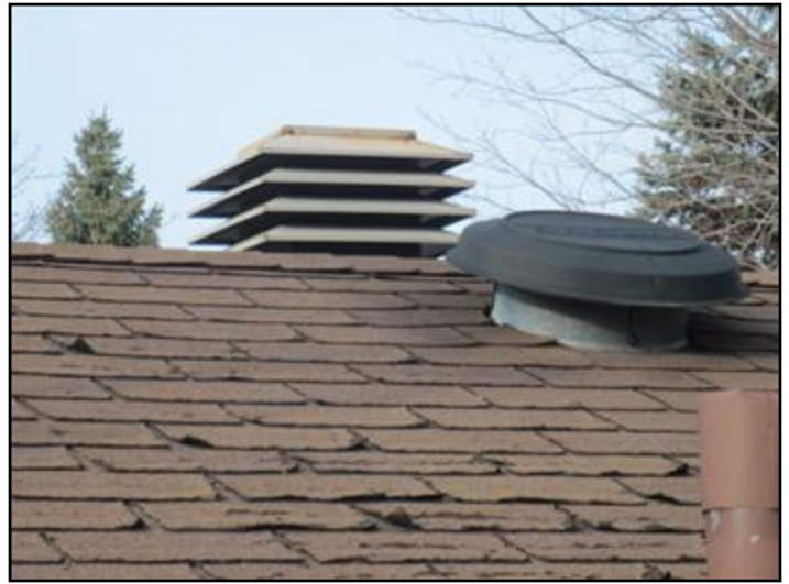
Roof shingles in poor condition
