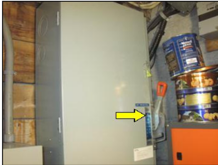
Main power disconnect
