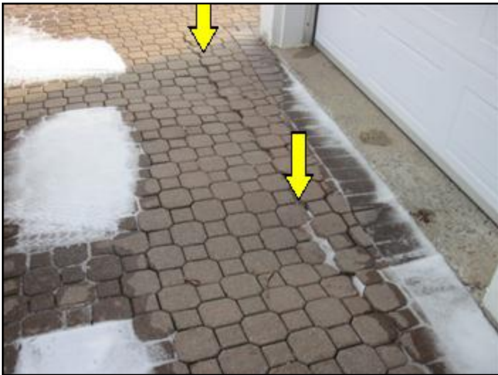
Excessive settlement in driveway
