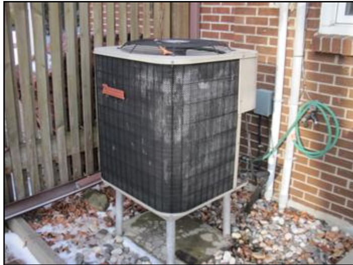
Heat pump condensing unit
