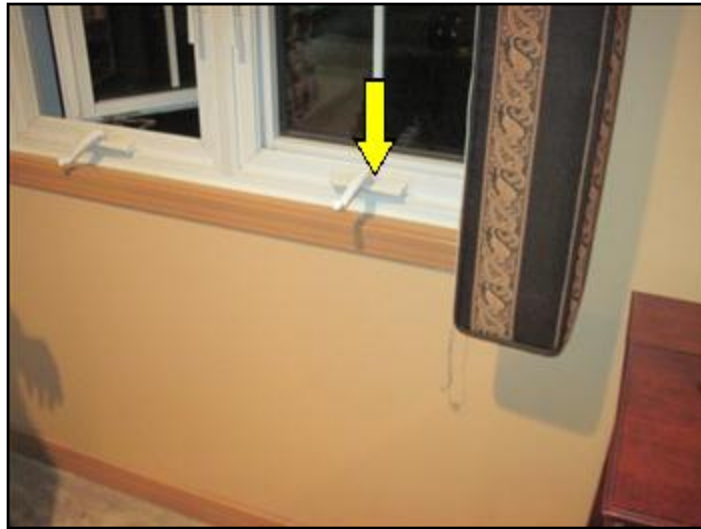
Damaged hardware in need of replacement
