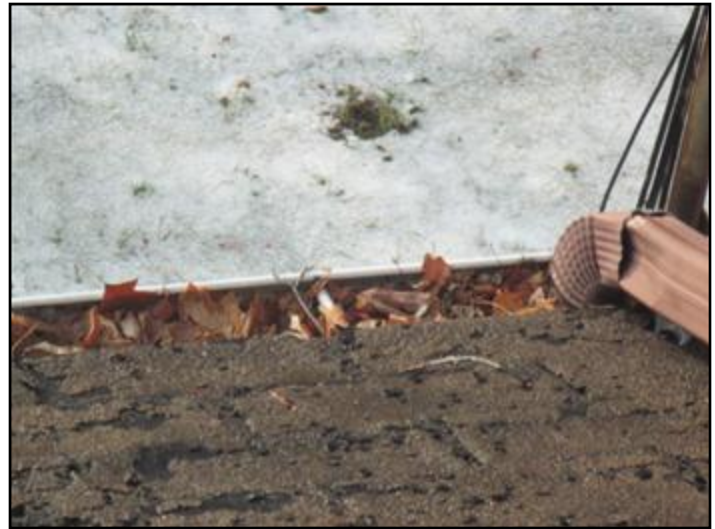
Rear gutter clogged and leaking
