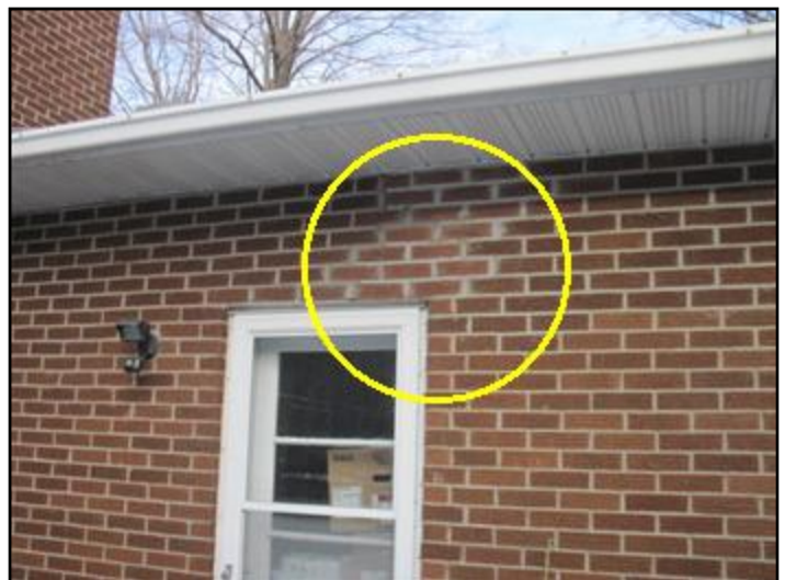
Crack in rear brick wall
