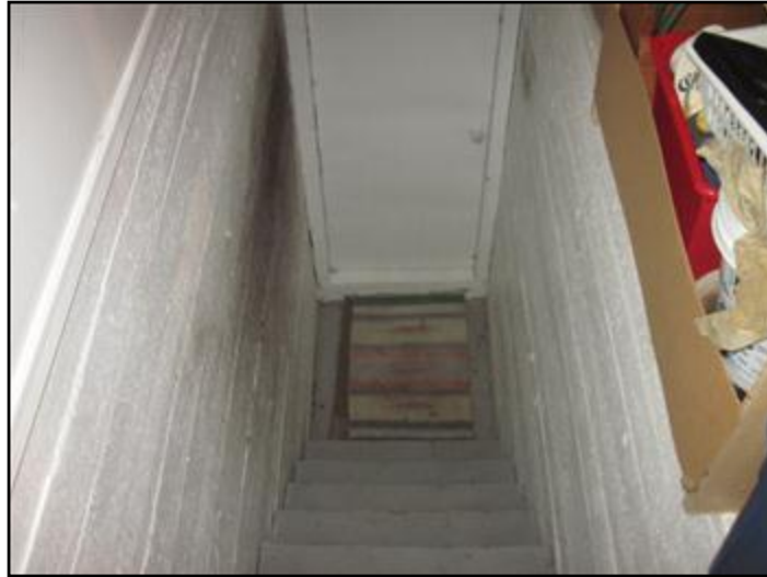
Handrail missing in staircase
