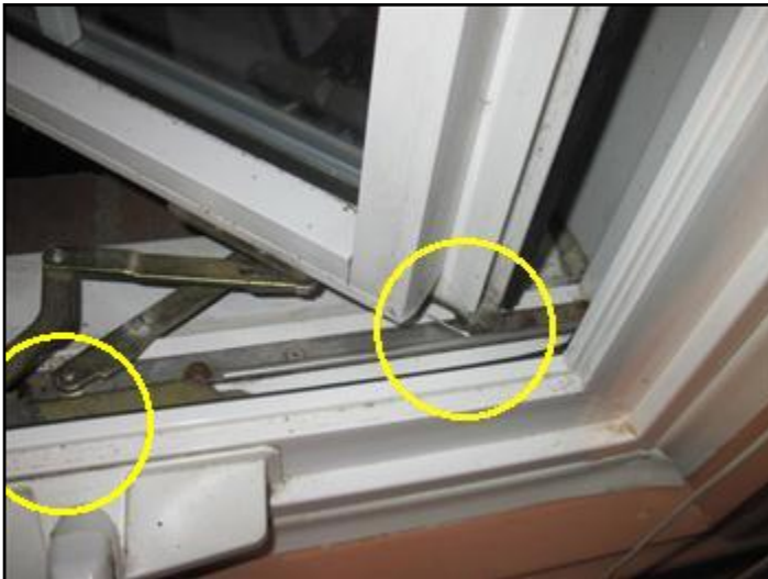
Damaged hardware in need of replacement
