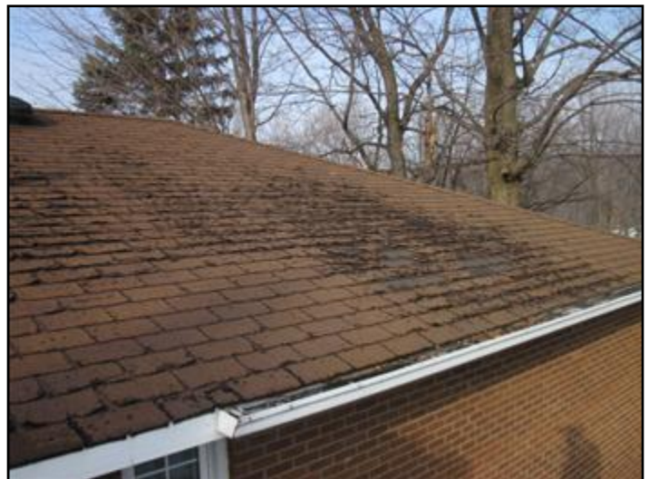
Roof shingles in poor condition
