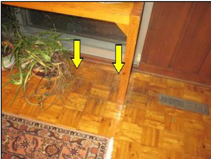
Water damage to floor covering
