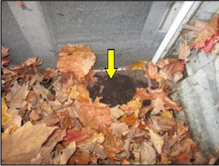
The ground is all the way up to the window
