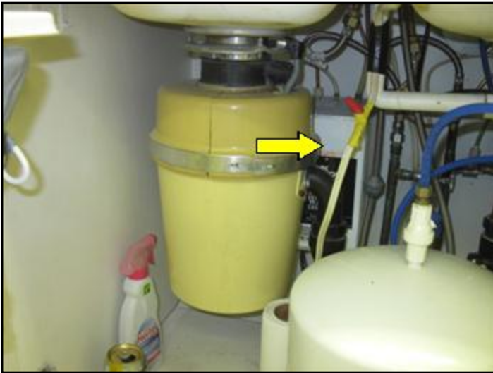
Improper electrical connection
