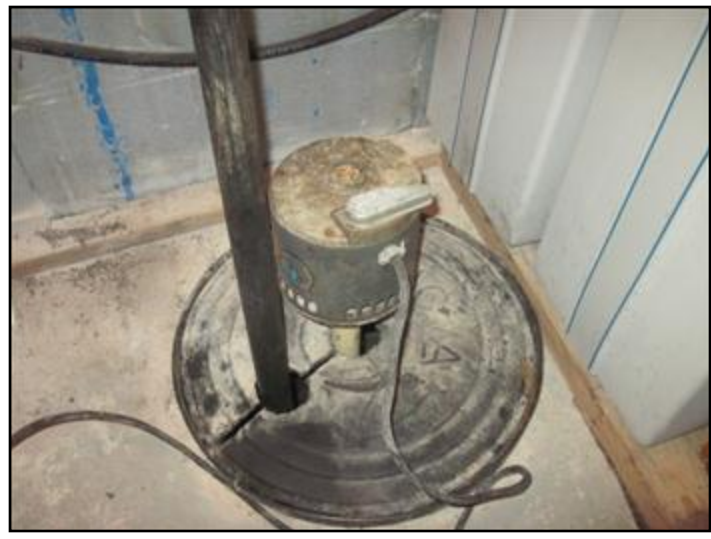
Sump pump not functional
