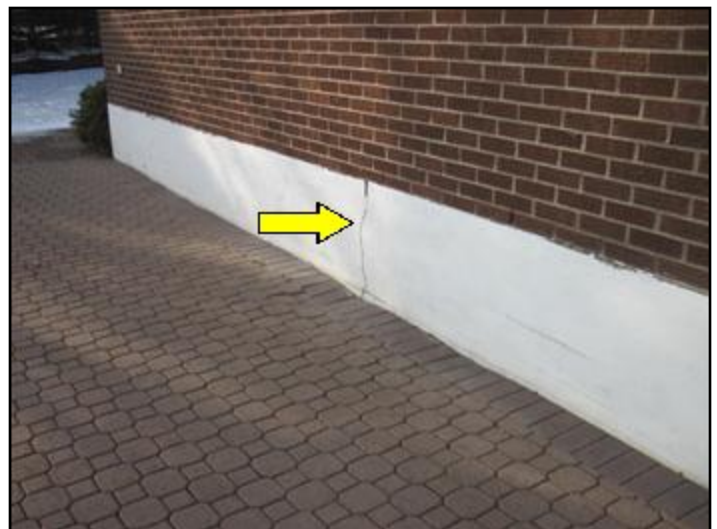
Crack in left side garage wall
