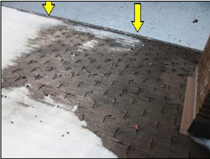
Rear gutter clogged and leaking
