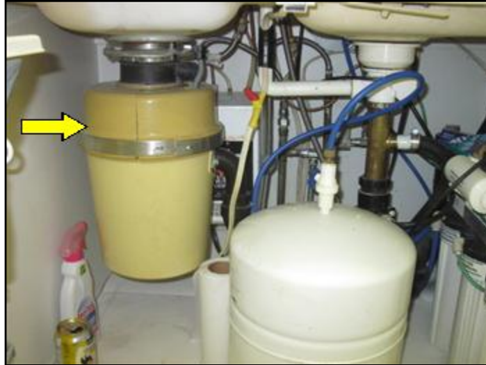
Garborator not functional
