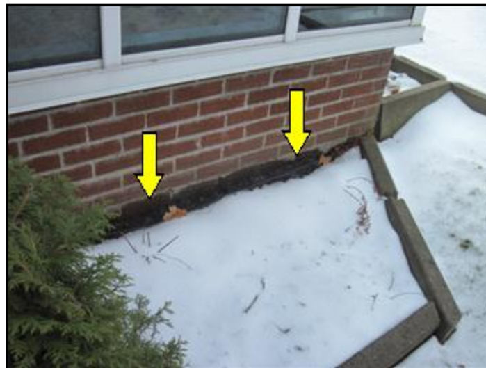
Masonry too close to grade
