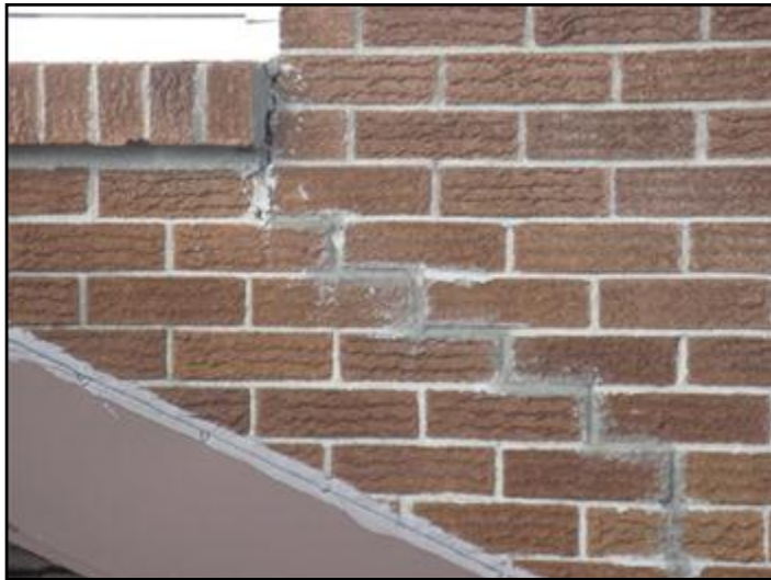
Crack in left brick wall second floor
