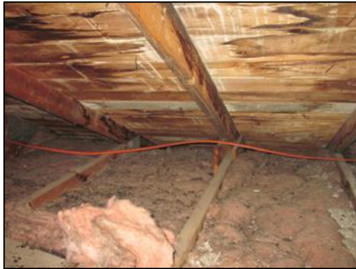
Limited insulation in garage attic
