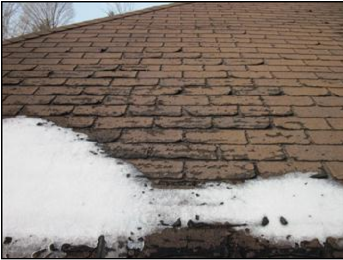
Roof shingles in poor condition
