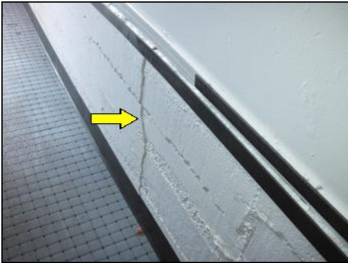
Left wall crack seen from inside
