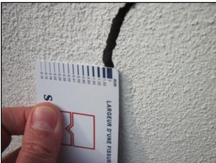
Crack in left wall exceeds 3mm
