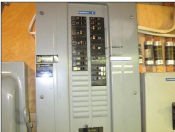
Square D breaker
