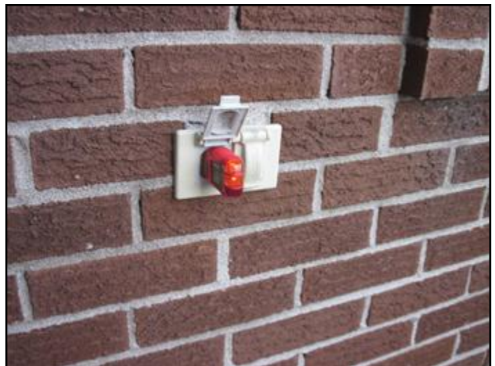
Exterior outlet missing GFI protection
