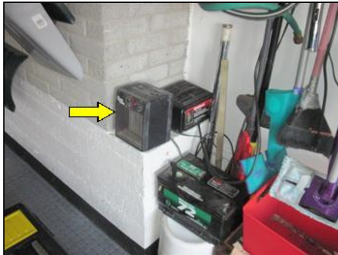
Heat source inadequate for the garage
