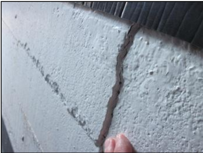
Approx 5mm of lateral displacement
