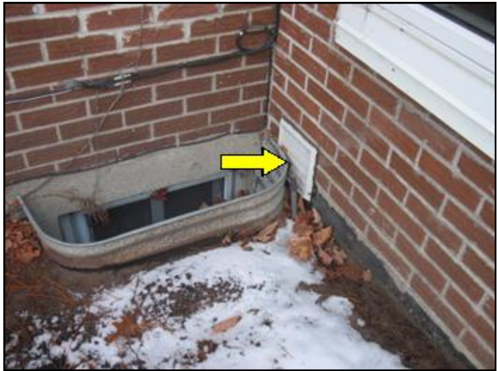
Bathroom vent hood blocked
