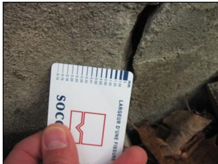
Crack in rear wall exceeds 3mm
