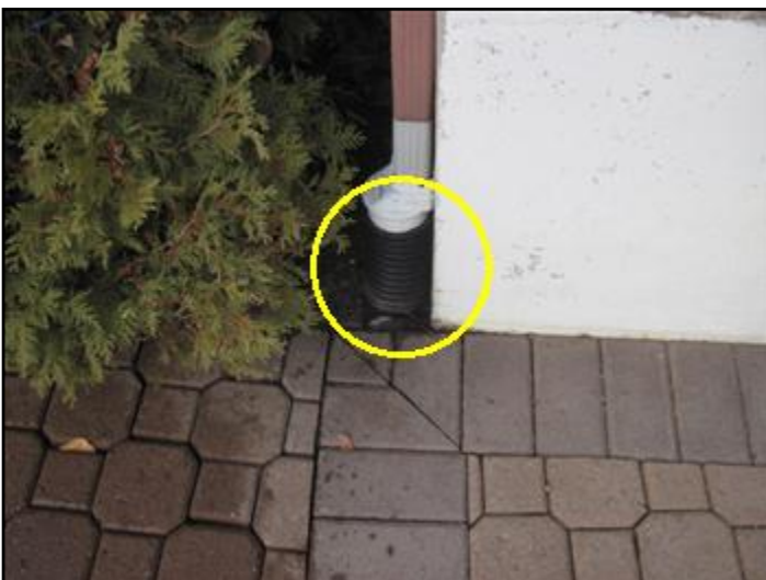
Perforated pipe used
