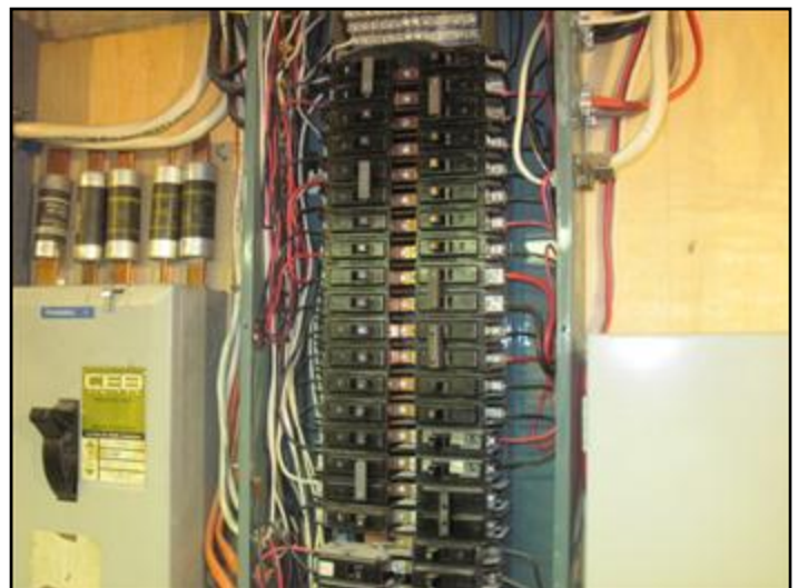
View inside CH panel
