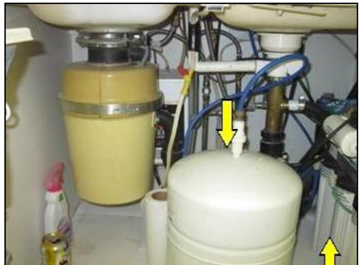
Water treatment system under kitchen sink
