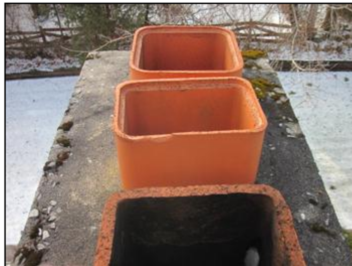
Rain caps and screens missing
