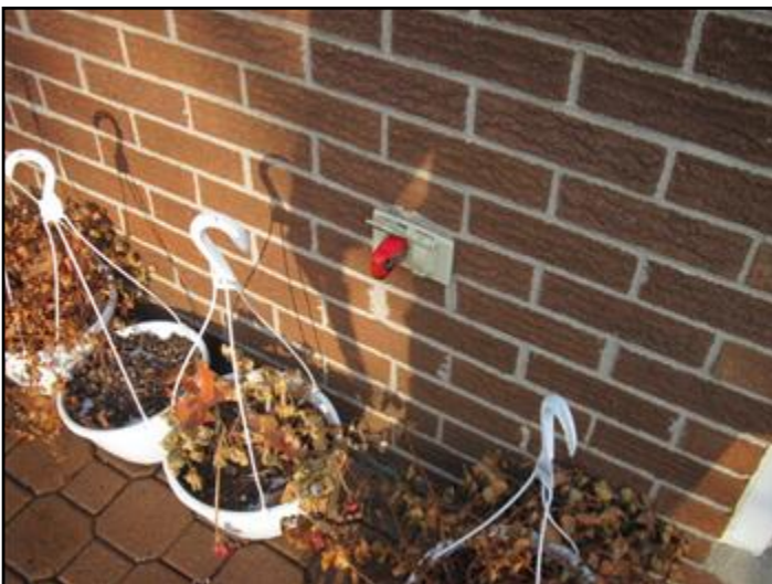
Exterior outlet missing GFI protection
