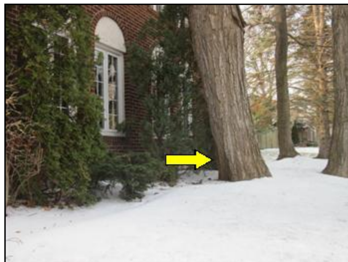
Large tree less than 2 metres from house
