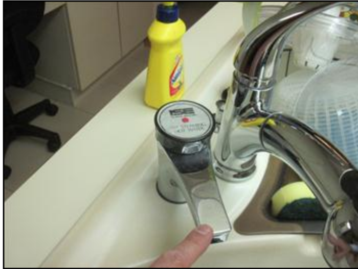
Hot water dispenser not functional
