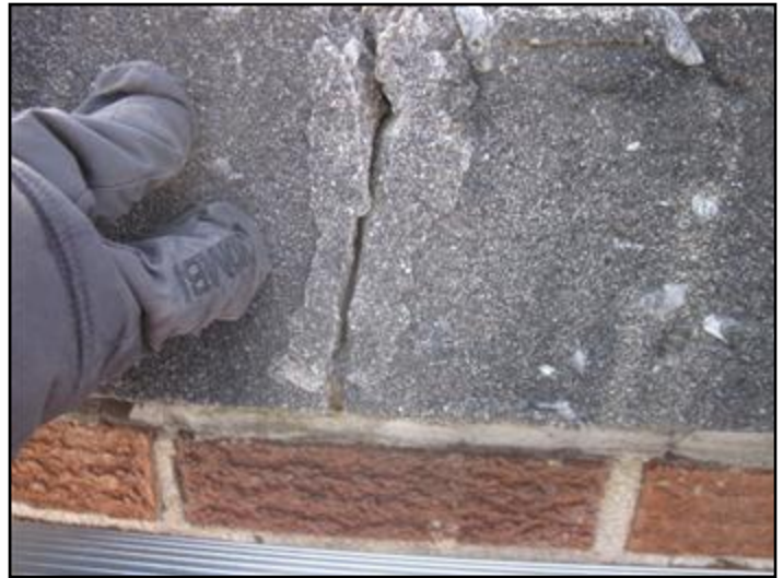
Chimney cap cracked
