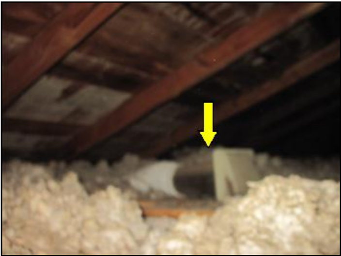
Inappropriate venting inside the attic
