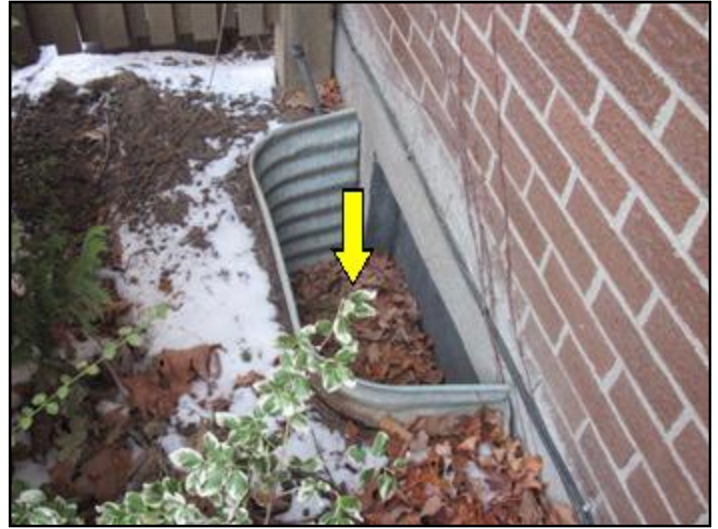
The ground is all the way up to the window
