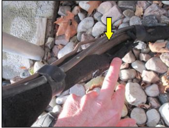
Exposed refrigerant line
