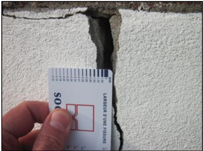
Crack in left wall exceeds 3mm
