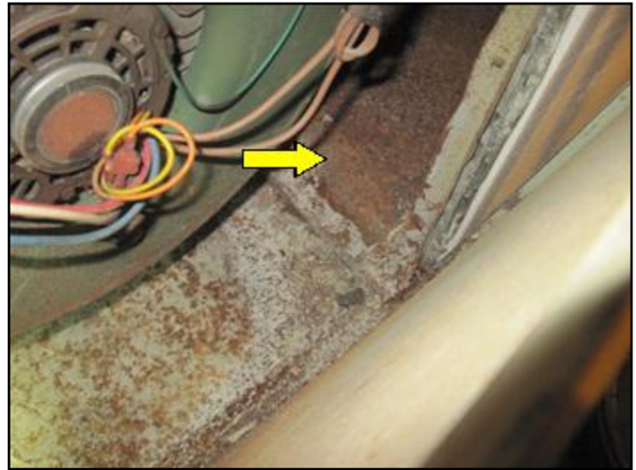
Rust inside furnace cabinet
