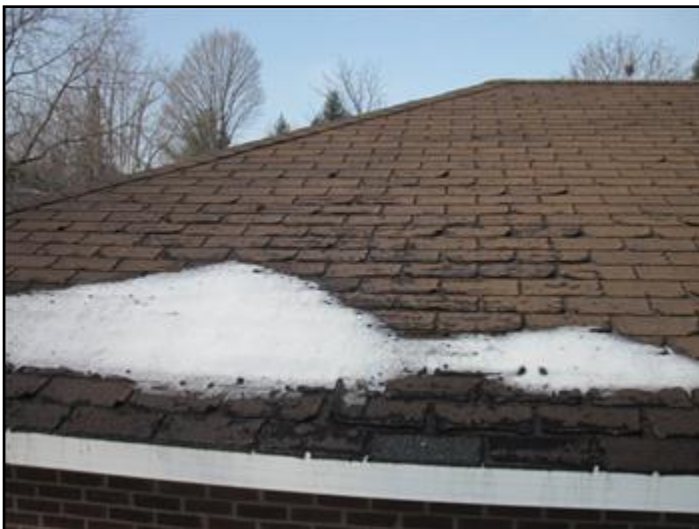
Roof shingles in poor condition
