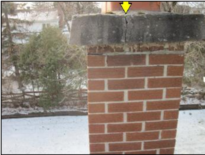
Chimney cap cracked
