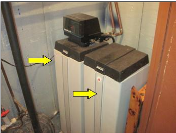
Water treatment system in basement
